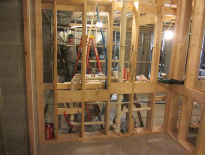
Plumbing and electric in the common wall between the toilets and kitchen.
