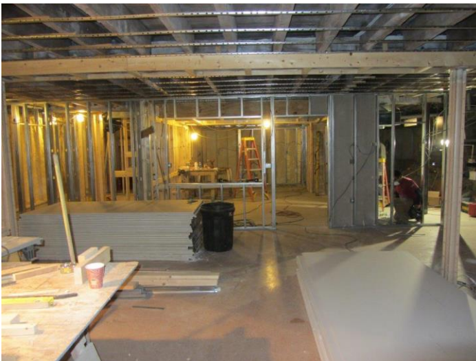
Standing at the back door looking toward the kitchen. Note the piles of sheetrock.
