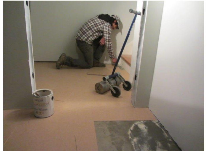
Cutting and gluing floor tile. The style and color match the existing tile.
