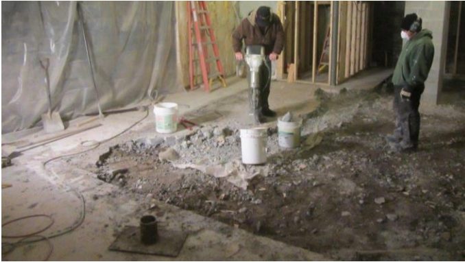
Jack hammering the uneven concrete floor. Broken concrete was carried out by hand.
