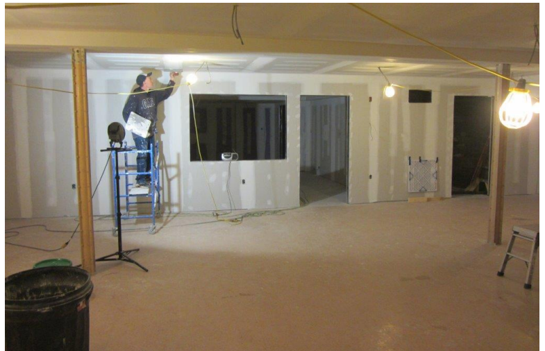
Standing at the back door looking toward the kitchen
