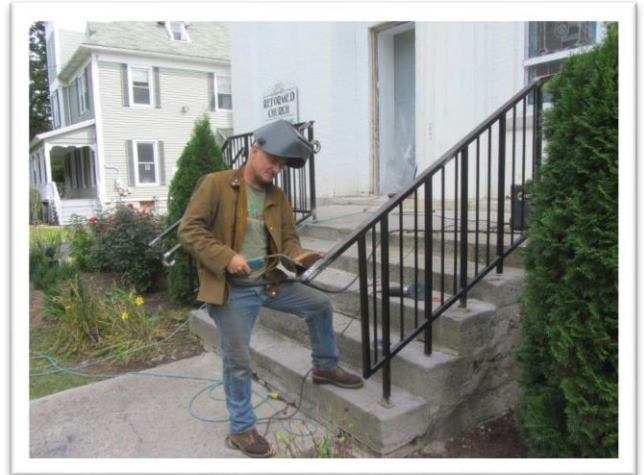
New railing is being installed. Safer. Much safer.
