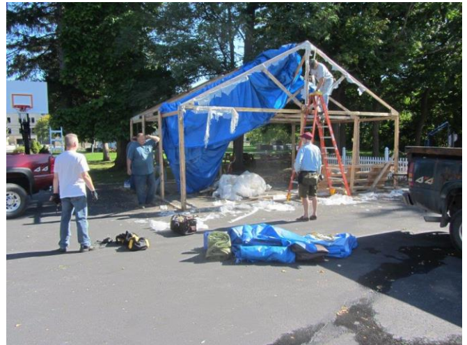
Disassembling the blue tent after finally removing the pews.
