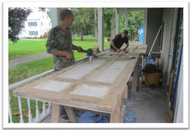
Sanctuary front doors being stripped and painted. They would not hold paint any longer – too many layers of incompatible coatings.
